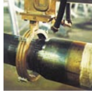
▲ Heat treatment for the weld zone
